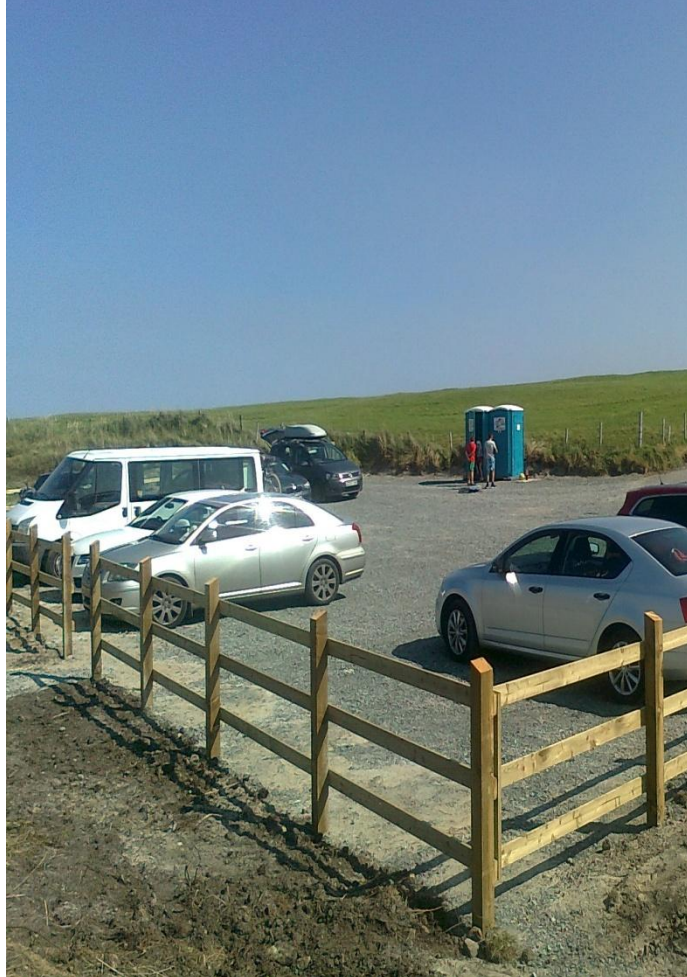
Dooley after maintenance works
